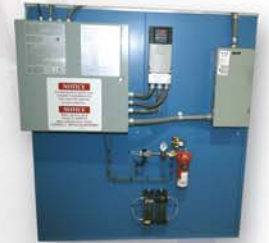
Prewired Control System Utilizing VFD For Pressure Control
