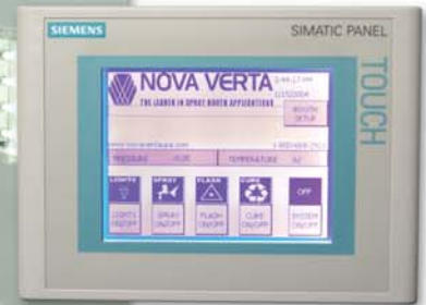
Siemens Touch Screen with Direct-Fired Systems
